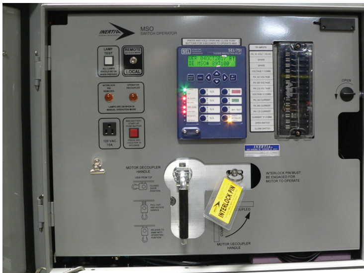
Control Panel of Inertia Motorized Switch Operator with SEL-751
