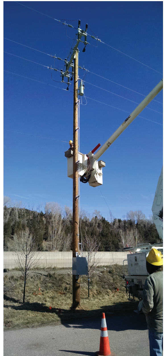
LineBOSS Underarm Configuration Switch Controlled by MacLean Motorized Switch Operator with SEL-751A
