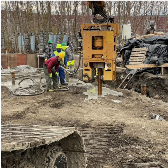
Grouted piles being installed to support large storage tanks:
