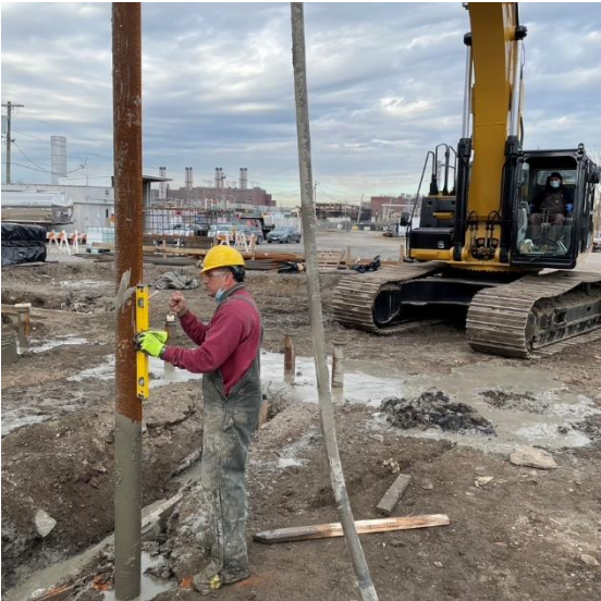
Grouted piles being installed to support large storage tanks:
