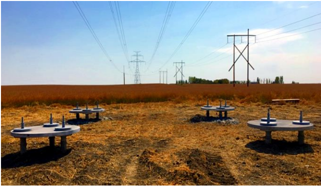
Grouted piles being installed to support large storage tanks:
